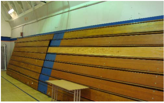
Need to replace gym bleachers.
