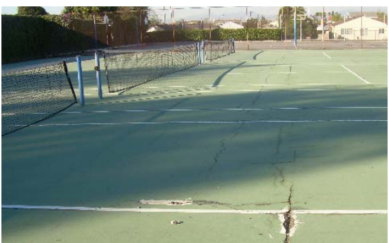
Tennis courts require resurfacing and/or replacing.
