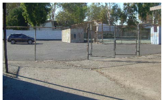
Major improvements are needed in security fencing.
