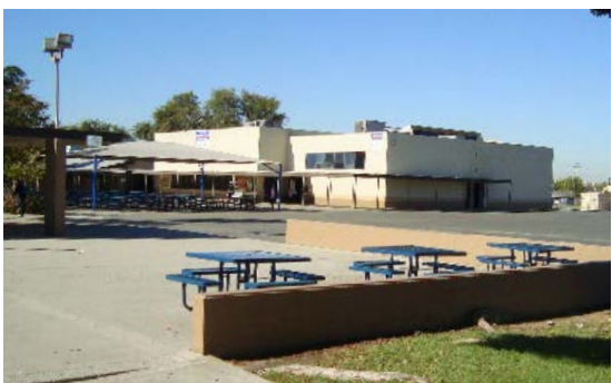
Lunch shelters need to be replaced/expanded.
