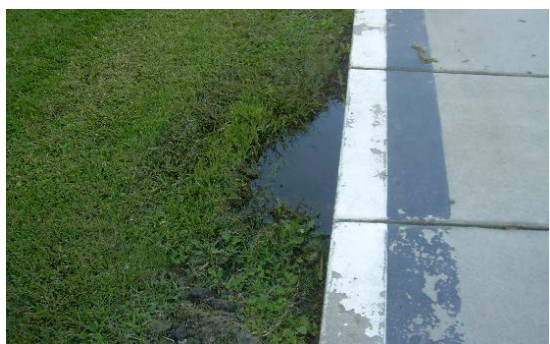
Address flooding/ponding issues between buildings.
